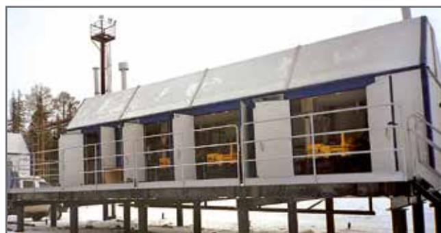
The process module is equipped with an automatic fire extinguishing system using aerosol generators.
